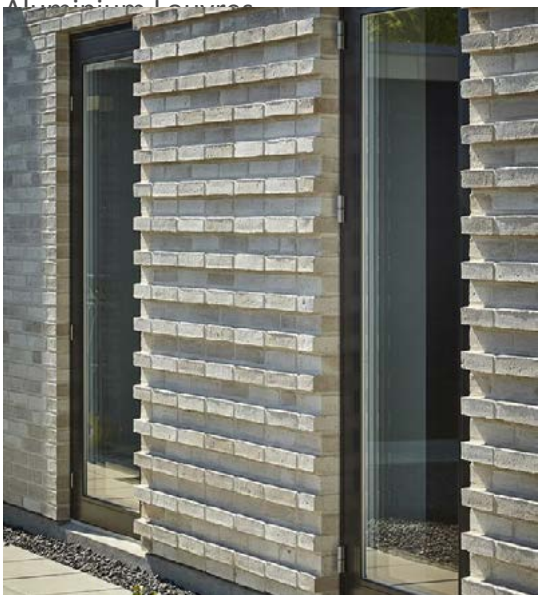
Protruding Brickwork - Detail 2
